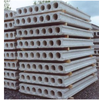
Figure 10: Typical hollow core slabs
